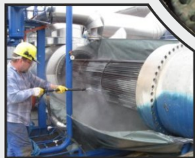
shell and tube heat exchanger
